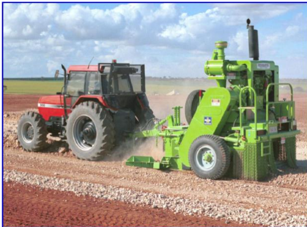
Figure 7 – Tractor towed 'Rockbuster' used to crush oversize material (Broons), Australia
